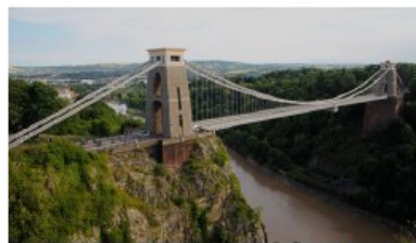
Clifton Suspension Bridge Bristol, England
