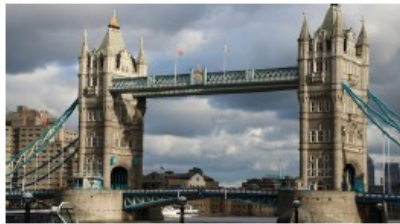
Tower Bridge London, England
